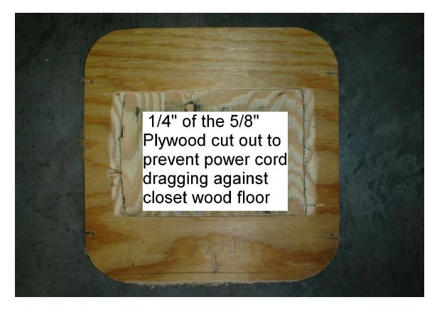
The above hatch cover is 5/8 inch thick plywood with carpet glued to the top of the plywood. The cover is recessed into the closet floor, when installed the cover disappears into the surrounding carpeted floor.
